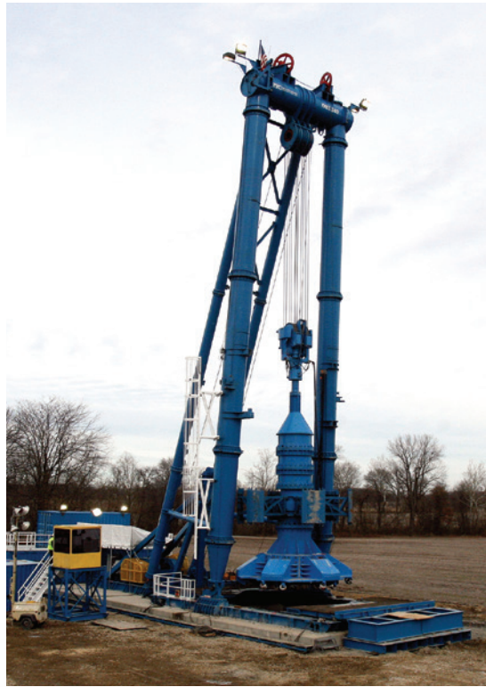
Left: 7 SP Raise Bore Machine setup in Manhattan, NY.
