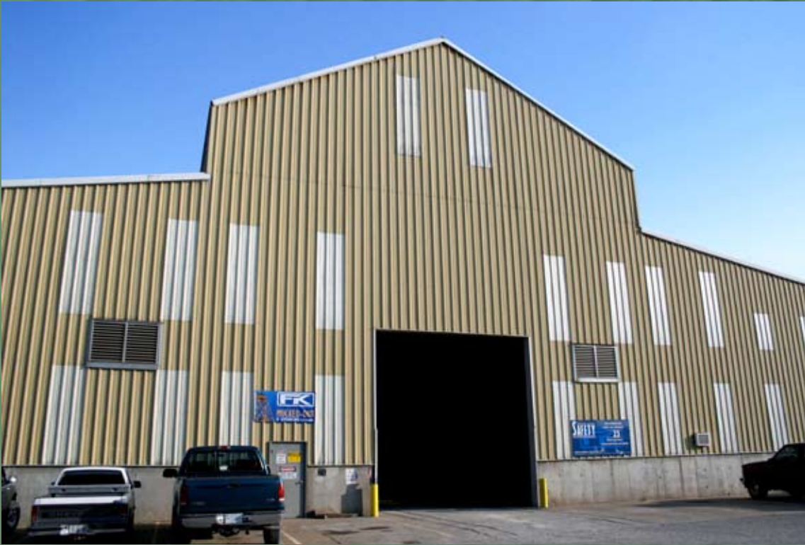
Frontier-Kemper's Shop facility, located at the Headquarters Office in Evansville, Indiana.
