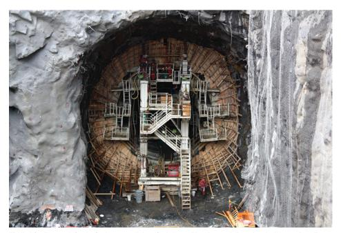
TRAIL, BC: Formwork for the final concrete lining of a Drill-and-Blast Penstock Tunnel at the Waneta Dam Tunnels project. [project on pg. 39]
