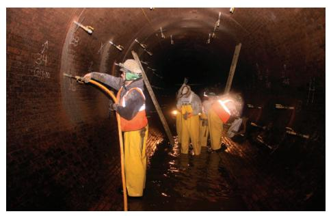
Rehabilitation of the New Croton Aqueduct-grouting behind the brick lining.
