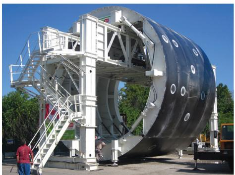
Inspection of the 7.5m walking, beam-style tunnel form designed to operate on a 17% slope.
