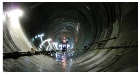
Inside one of the penstock tunnels during placement of the cast-in-place, concrete liner.
