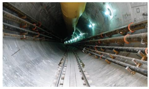
Tunnel A lined with precast concrete segments-with track in invert and utilities hung from the walls.
