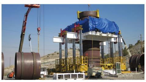
The fully operational Gantry System lowering a welded, steel can into the NVR.
